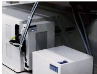
Main control box
